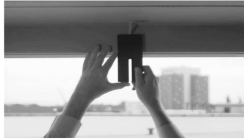
Align the mounting bracket on the top lintel at the center of the doors. With the mounting bracket installed, attach EyeSeal Unit to the mounting bracket using the bolt and the washer. Adjust the EyeSeal Unit until the top of the unit is seated against the lintel.
